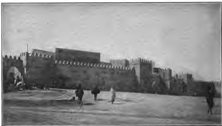
FIG. 242.—Wall around Sfax, Tunis, built as a defense against the desert nomads before they were reduced to order by the French.
